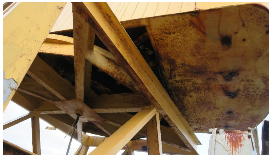
Kranhuset sett under.
