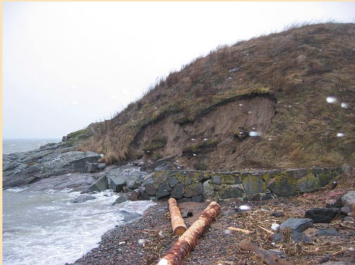
Figures 6 and 7. Damage at the Suomenlinna Fortress caused by sea level rise in January 2005. Left: Gun battery on Länsi-Mustasaari Island with collapse of its supporting wall and sand earthworks caused by high sea level and waves (Photo: Heikki Lahdenmäki, Suomenlinna Governing Body). Right: Shoreline wall on Pikku-Mustasaari Island with erosion caused by high sea level and waves (Photo: Heikki Lahdenmäki, Suomenlinna Governing Body).
